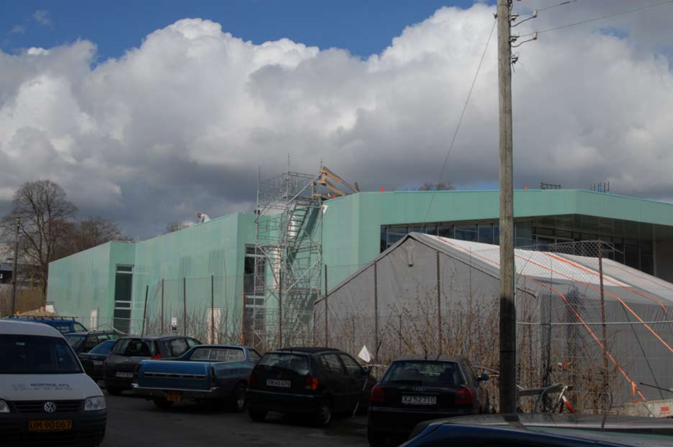
Ordrup Library and sport facilities , in collaboration with NORD - under construction
